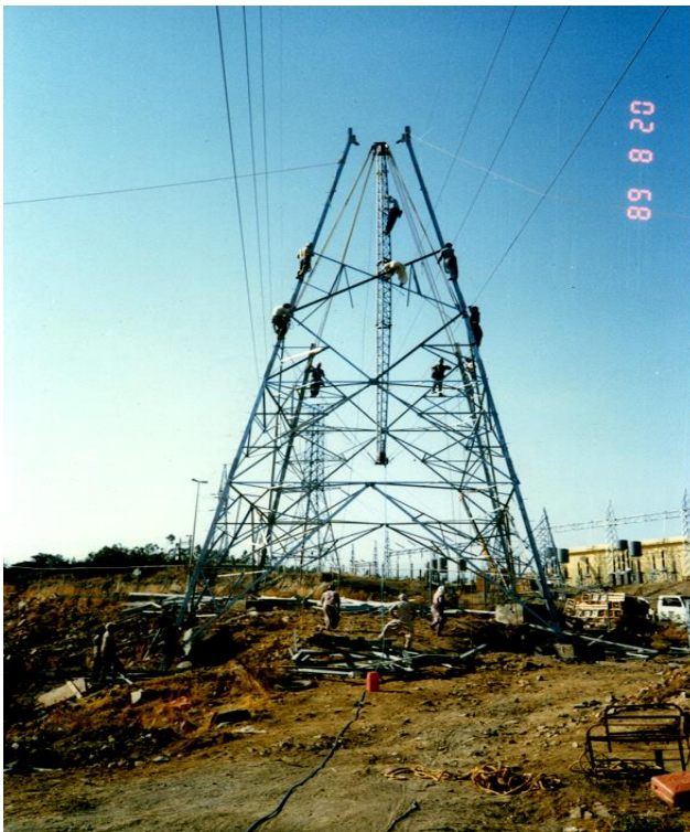
TOWER ERECTION OF 132kV DOUBLE CIRCUIT TRANSMISSION LINES AL-BAHA (SUADIA) Stringent Procedures of Tower Erection Various Activities by Gin Pole Method in one of the most difficult hilly terrain of the Southern region of Saudi Arabia (1989) – By GEM SEEROO
