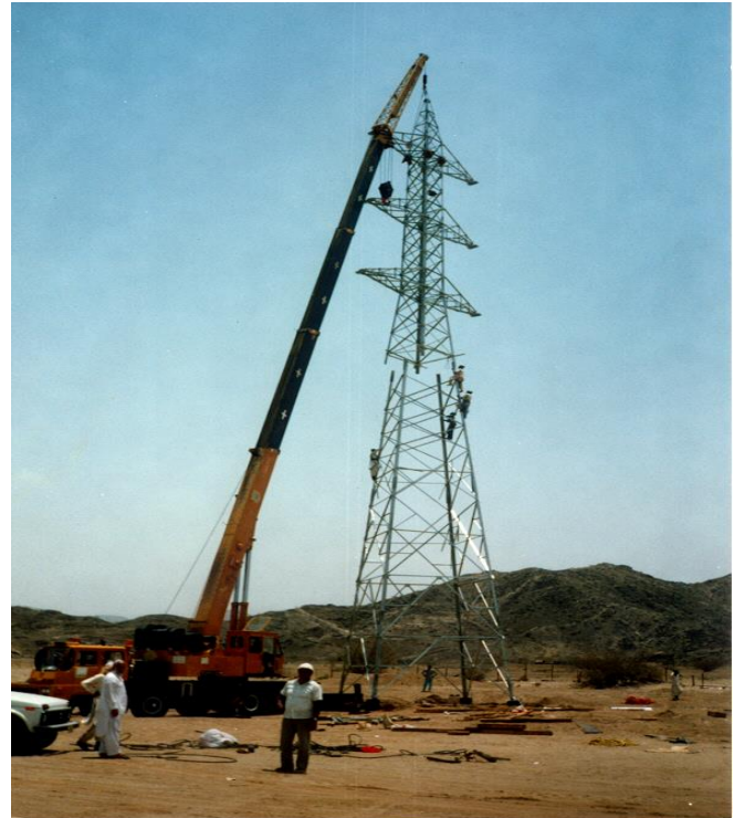
DIVERSION OF 110kV DOUBLE CIRCUIT O.H. TRANSMISSION LINES AT ARAFAT – MAKKAH Tower Erection Works by 60 Ton Telescopic Crane in Progress (1992) - BY GEM SEEROO
