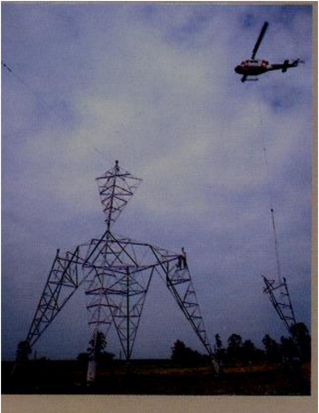
TOWER ERECTION WORKS CARRIED-OUT BY VARIOUS STRINGENT PROCEDURES ARE IN PROGRESS 500kV DOUBLE CIRCUIT OVERHEAD TRANSMISSION LINES (1996 - 97) JUNGONG - GURUN (Line-4, SUMITOMO Japan) AT MALAYSIA - BY GEM SEEROO
