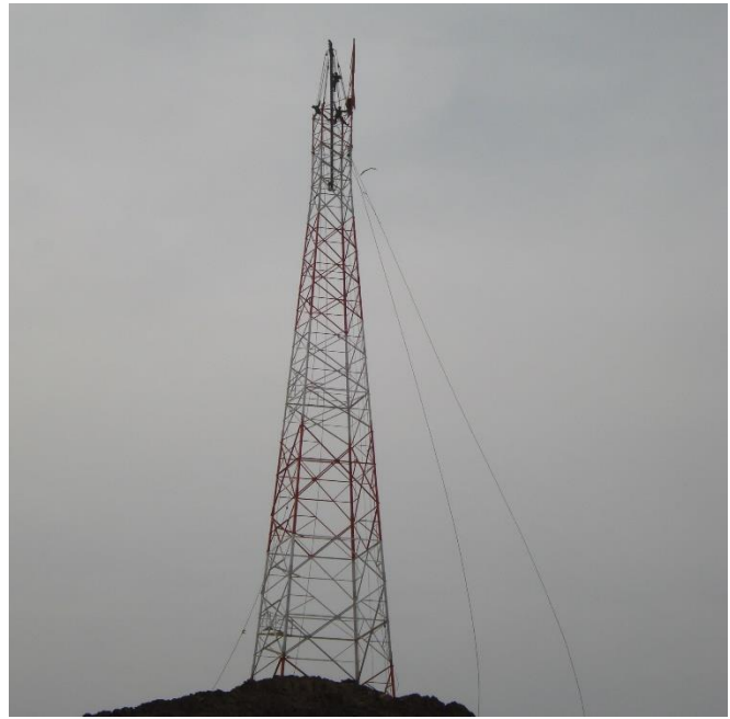
VARIOUS ERECTION STAGES BY GIN POLE METHODS ADOPTED FOR STC GSM TOWER ZBH 924R11 AT JAREEN VILLAGE – SAUDI ARABIA, BY GEM SEEROO WITH THE JOINT COLLABORATION OF EWACO IN 2007
