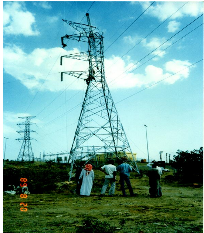
TOWER ERECTION OF 132kV DOUBLE CIRCUIT TRANSMISSION LINES AL-BAHA (SUADIA) Stringent Procedures of Tower Erection Various Activities by Gin Pole Method in one of the most difficult hilly terrain of the Southern region of Saudi Arabia (1989) – By GEM SEEROO
