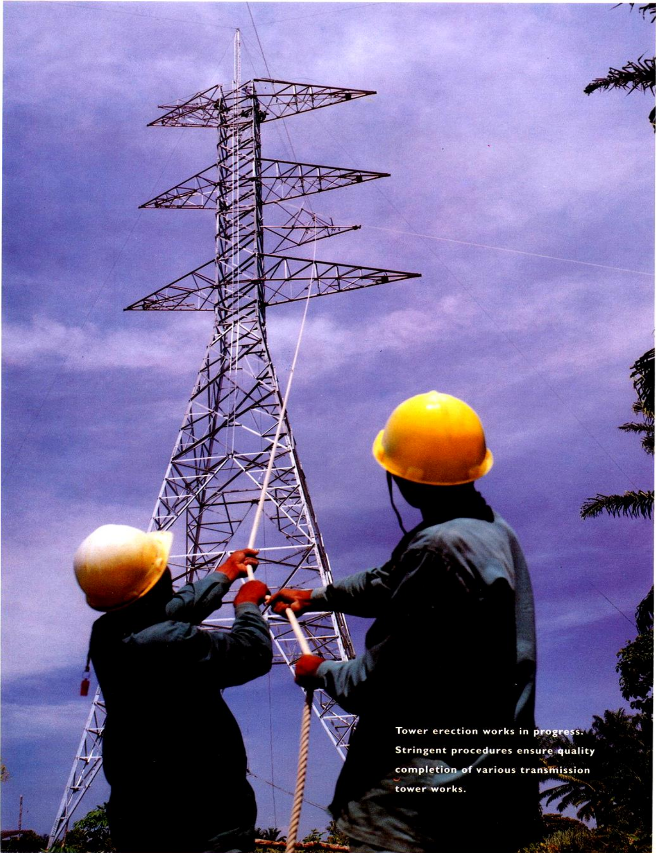
Tower Erection By GIN Pole Method 500kV DOUBLE CIRCUIT OHTL Malaysia (1996 - 97) JUNGONG - GURUN (Line-4, SUMITOMO Japan) AT MALAYSIA - BY GEM SEEROO
