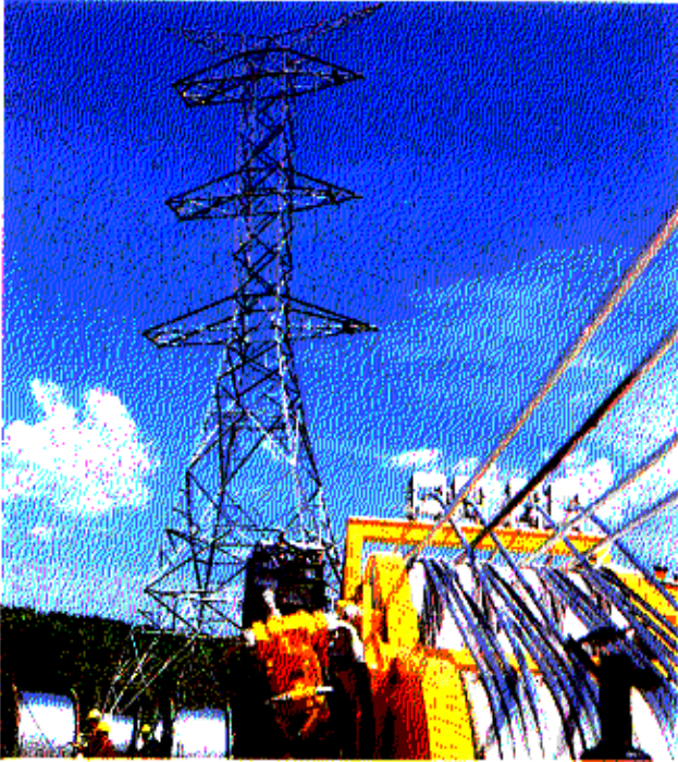
VARIOUS STAGES OF QUAD - BUNDLED CONDUCTORS STRINGING IN PROGRESS 500KV DOUBLE CIRCUIT OHTL (1997 - 98) JUNGONG - GURUN (Line-4, SUMITOMO Japan) AT MALAYSIA - BY GEM SEEROO
