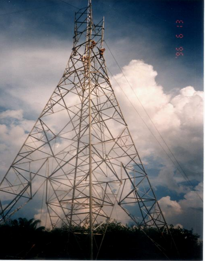
TOWER ERECTION WORKS CARRIED-OUT BY VARIOUS STRINGENT PROCEDURES ARE IN PROGRESS 500kV DOUBLE CIRCUIT OVERHEAD TRANSMISSION LINES (1996 - 97) JUNGONG - GURUN (Line-4, SUMITOMO Japan) AT MALAYSIA - BY GEM SEEROO
